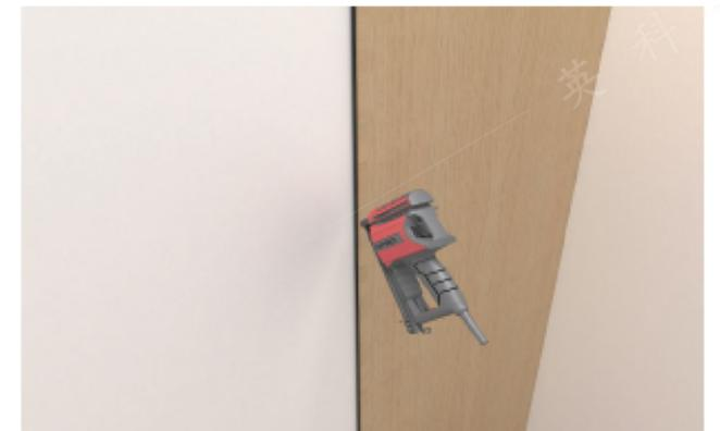
4. Insert the metal trim into the groove from the side of the panel, and then nail the metal trim to the wall.
